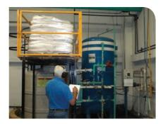
Smiths Interconnect EMC Technologies in Costa Rica was one of Smiths Group's largest water users. As part of its water reduction efforts, it installed a water recycling system on the sputter-wrap process. This reduced water use by more than 1,550 cubic metres per year, or 13%.
