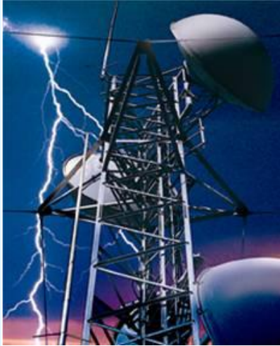
Telecoms lightning strike protection
